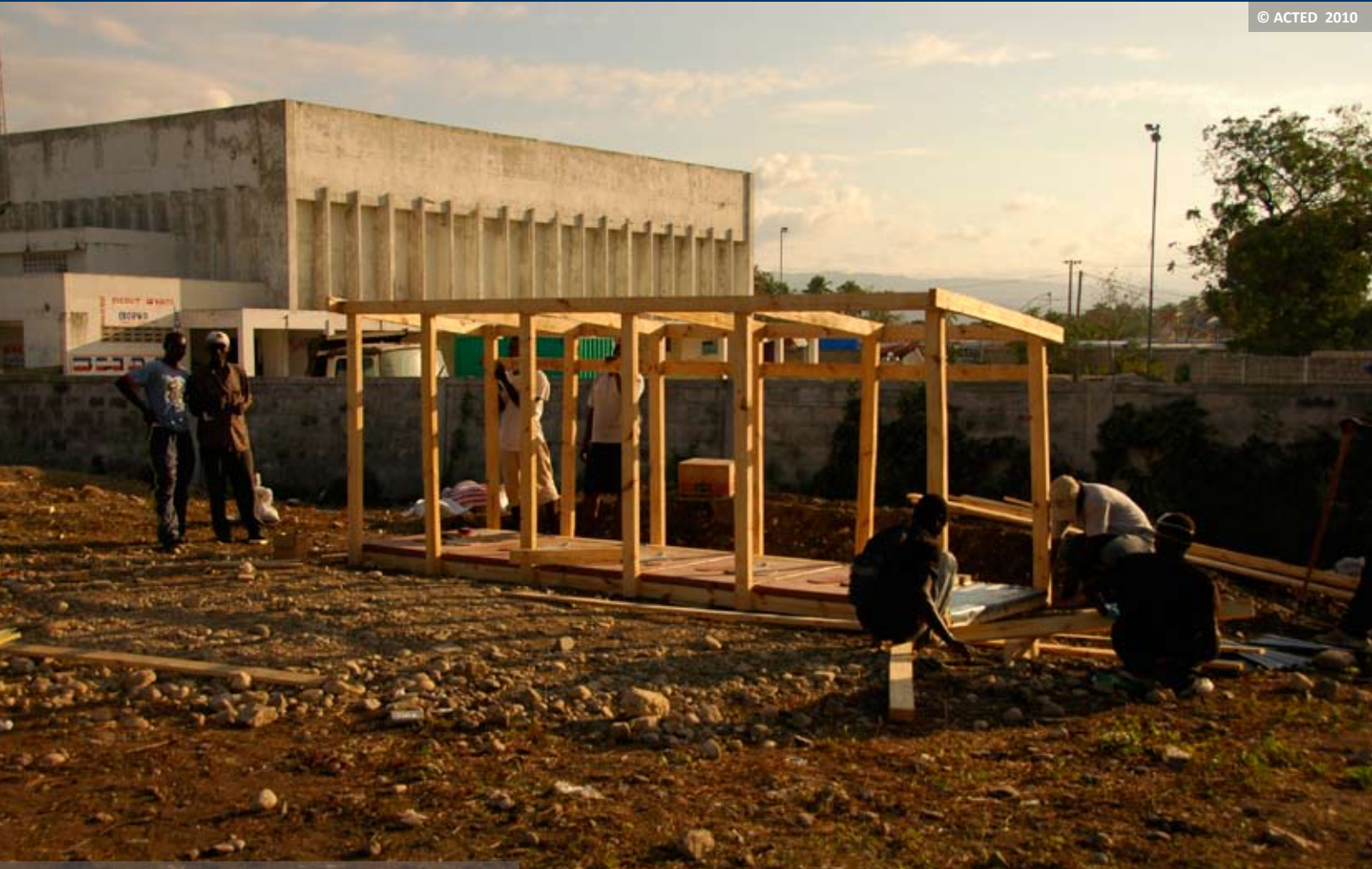
Setting up of latrines in the spontaneous settlement of Leogane. Construction de latrines dans un rassemblement informel de Léogane.
